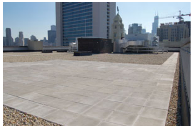
Photo 4: Ballast coverage of 17 pounds per square foot or greater and concrete pavers provide greater benefits than cool roof membranes.
