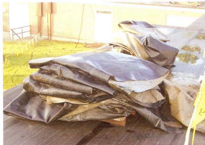
EPDM membrane pieces before they are transported to a grinding facility
