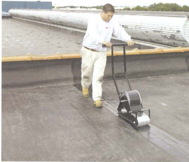
Improvements made in technologies for seaming, flashing and securement also have contributed to an impressive decline in maintenance costs.
